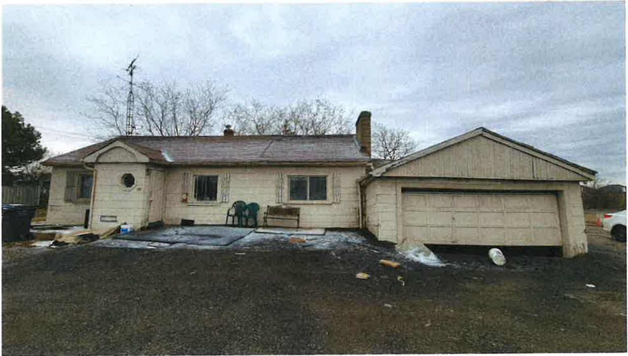
Front view of residential structure located in the northern portion of the subject site (looking southeast)
