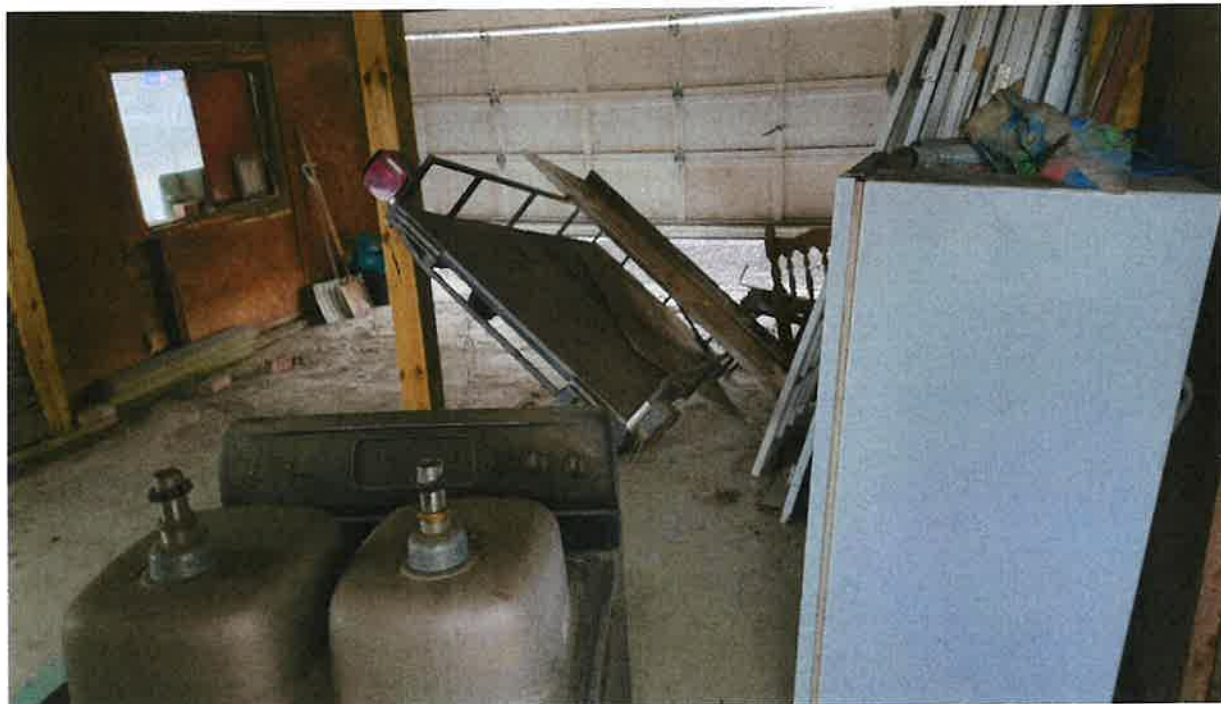
Inside view of the attached car garage in the northern portion of the subject site
