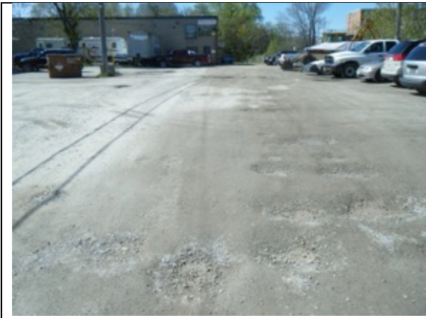
IMAGE 1 ASPHALT AND GRAVEL DRIVEWAY
