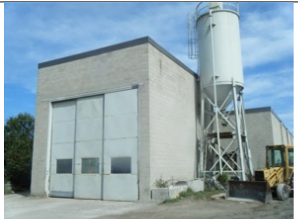
IMAGE 18 STRUCTURE AND SILO
