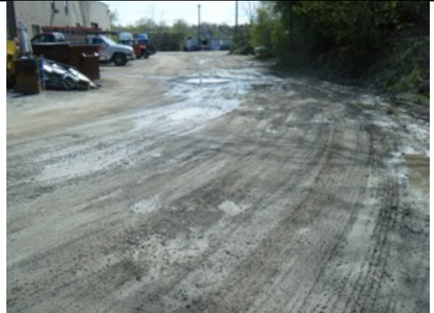
IMAGE 10 ASPHALT AND GRAVEL AREA
