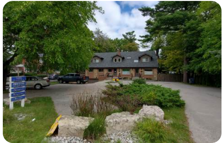
1495 Hurontario Street looking east
