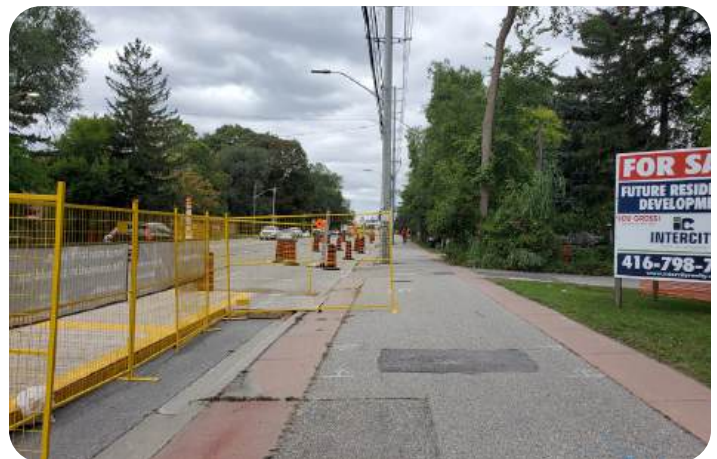
Subject Site frontage along Hurontario Street
