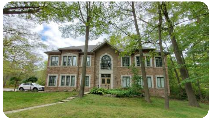
1470 Hurontario Street looking south from Indian Valley Trail
