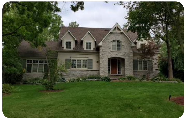
39 Pinewood Trail looking north
