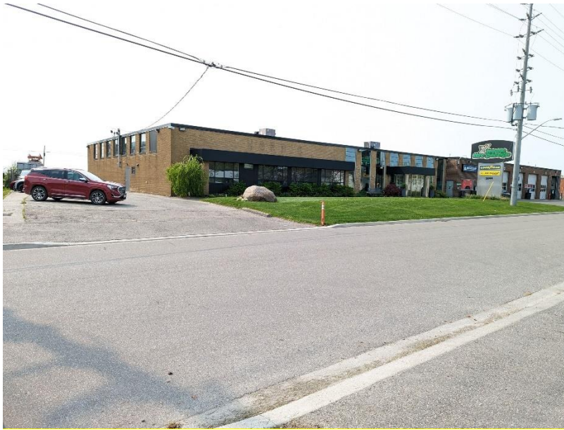
Image 17: View of 1044 Rangeview Road.
