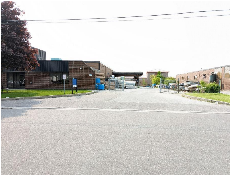
Image 36: View of the southwest side of 880 Rangeview Road.
