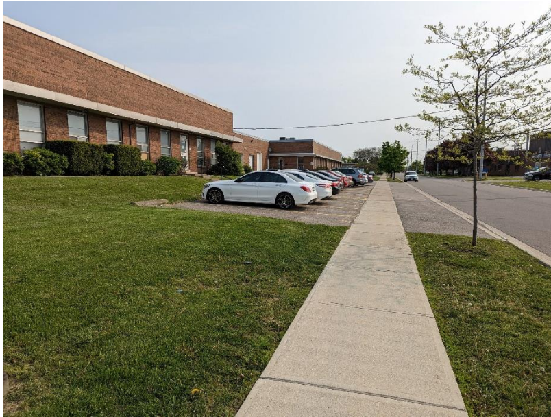
Image 37: View of the southeast side of 851-865 Rangeview Road.
