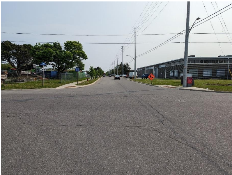
Image 30: View northeast along Rangeview Road from the intersection with Lakefront Promenade.
