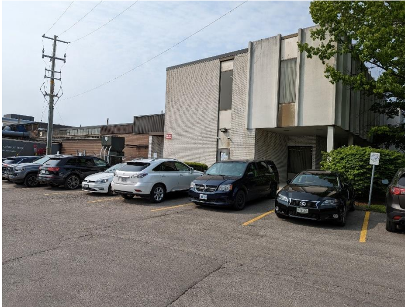
Image 9: View of the structure at 1000-1006 Lakeshore Road East.
