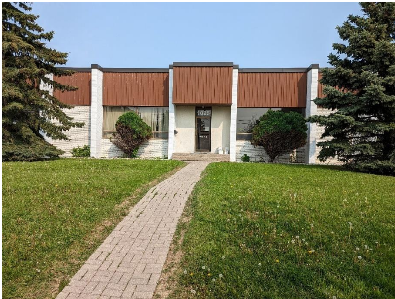
Image 22: View of 1025 Rangeview Road.
