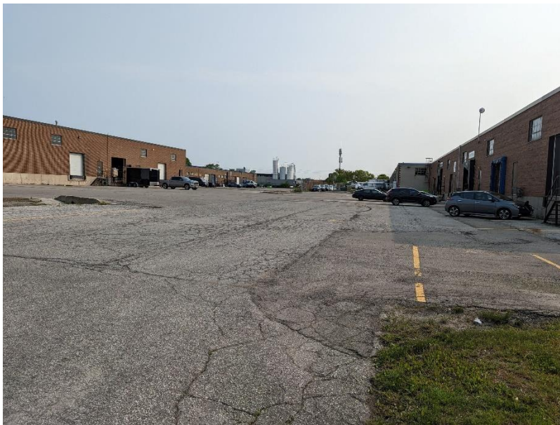
Image 38: View of the rear of 851-865 Rangeview Road.
