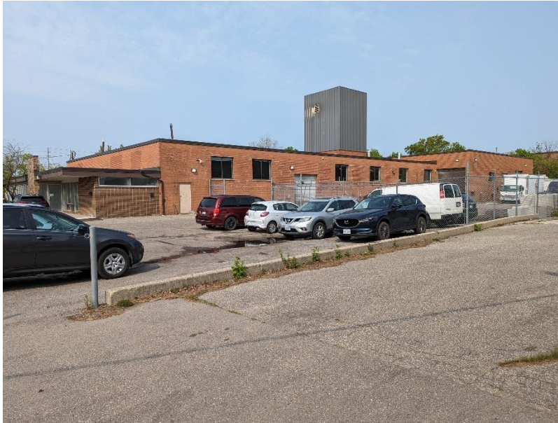
Image 25: View of 983 Rangeview Road.
