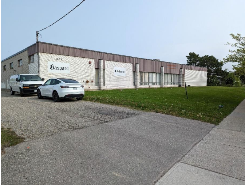
Image 19: View of 1035 Rangeview Road.
