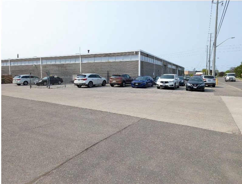
Image 29: View of 895 Lakefront Promenade at the south-central limit of the project area.
