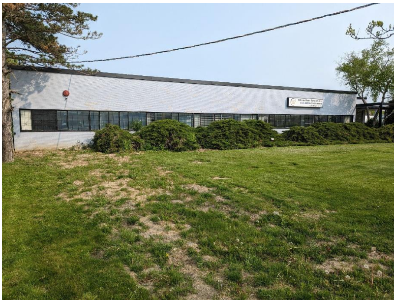
Image 18: View of 1045 Rangeview Road.
