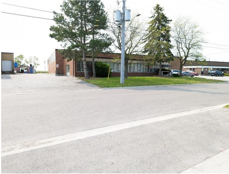
Image 23: View of 996 Rangeview Road.
