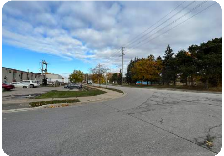
View of Hydro Road looking north.
