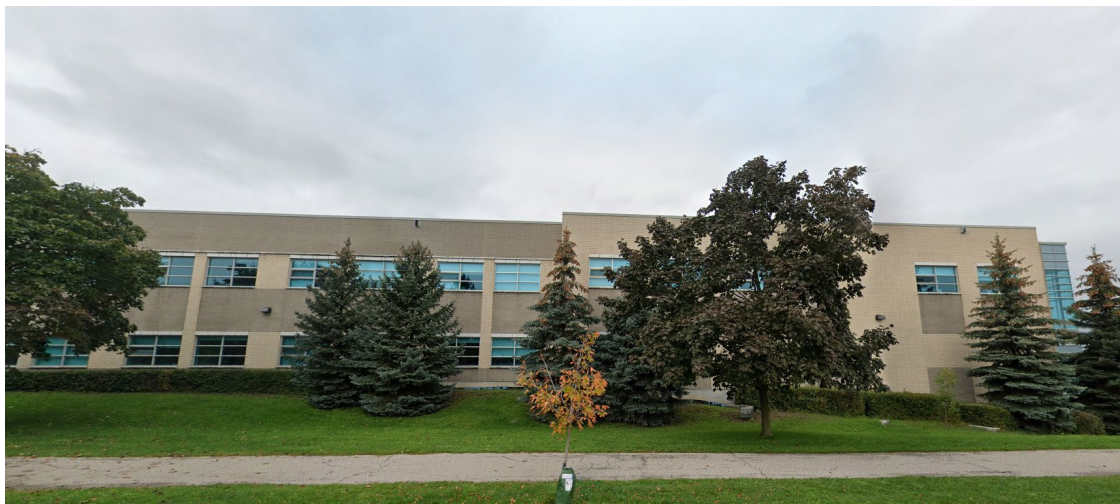
Figure 13. Surrounding Built Form: John Cabot Catholic Secondary School along Rathburn Road East (Looking Northwest)
