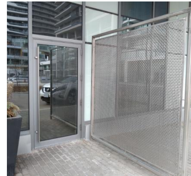
Image 4: Examples of wind control measures applicable to the secondary entrance
