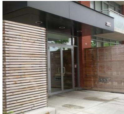
Image 4: Examples of wind control measures applicable to the secondary entrance
