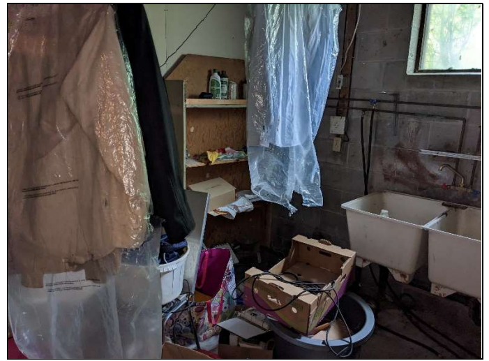
8. View of the other side of the boiler room.
