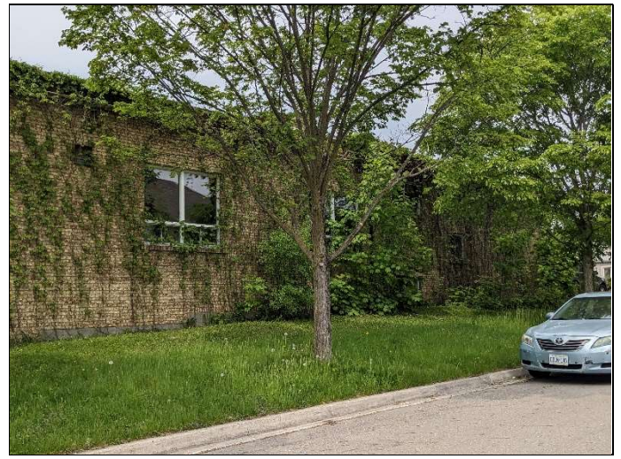
2. East side of the on-site dwelling, facing northwest.
