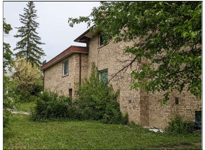
4. View of the west side of the on-site dwelling, facing northeast.
