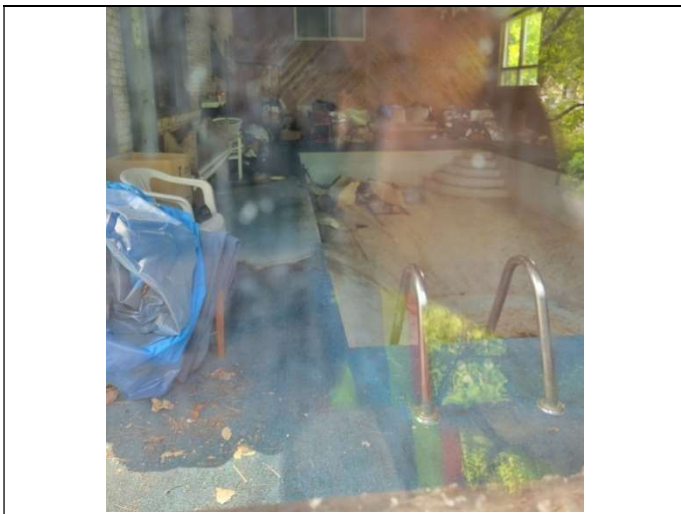
9. View of an indoor pool, backfilled with concrete, located on the southeast portion of the on-site dwelling.
