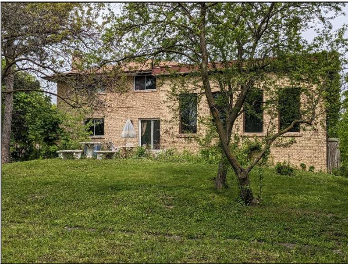
3. View of the south side of the on-site dwelling, facing north.
