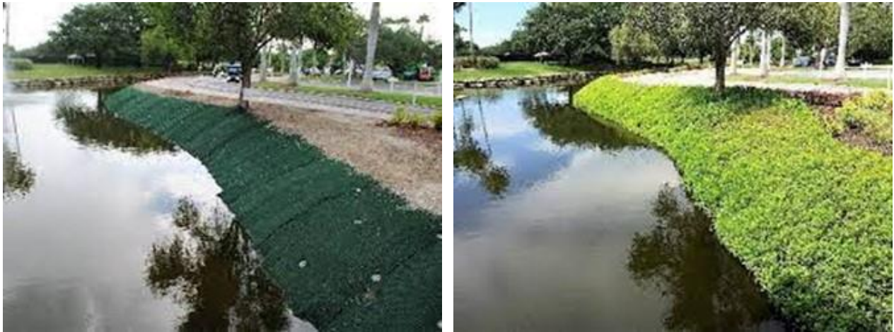
Figure 6-2: Non-Structural Bank Protection
