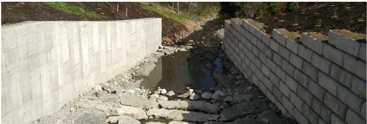
Figure 6-1: Structural Slope/Bank Protection (Armourstone Retaining Wall)
