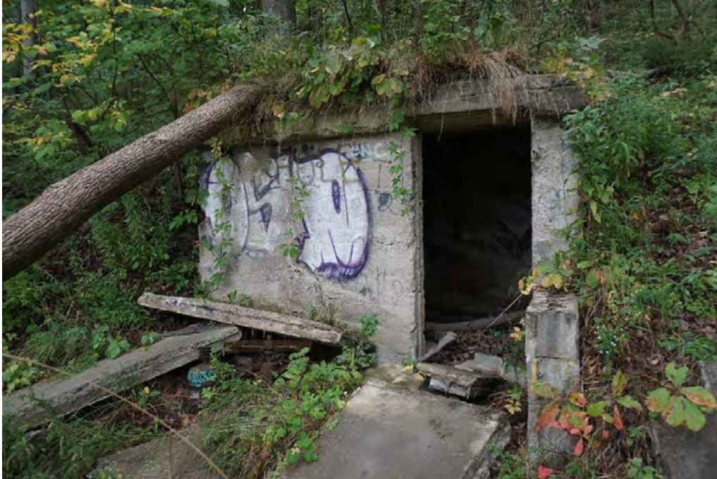
Photograph 14: View of the small concrete utilitarian building located in Study Area 2, presumed to have served as a pumphouse and the scattered scrap metal and machinery, looking east (AECOM 2023)
