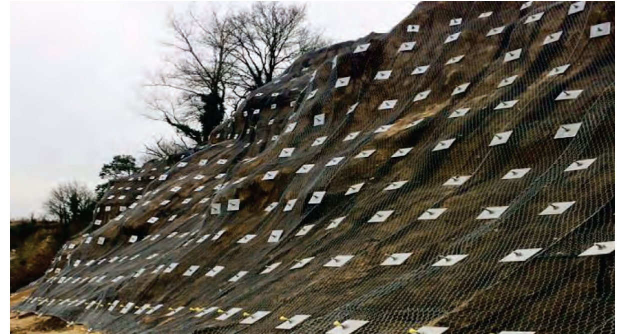
Example of Structural Bank Protection – Soil Nails
