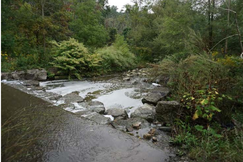
Photograph 10: View of Wolfedale Creek located in Study Area 2, the armour stone/concrete retaining wall and the surrounding low-lying riparian area, looking east (AECOM 2023)
