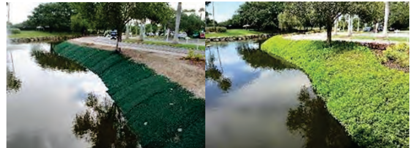
Example of Non-structural Bank Protection – Turf Reinforcement Matting
