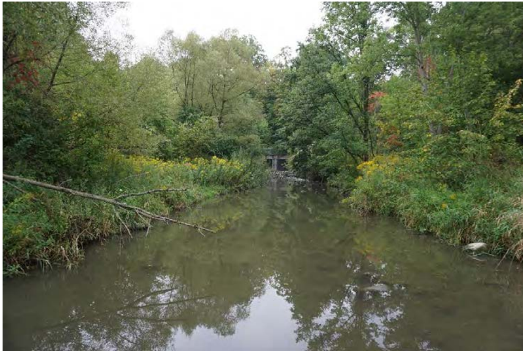
Photograph 12: View of Wolfedale Creek located in Study Area 2, a concrete engineered culvert and the surrounding low-lying riparian area, looking north (AECOM 2023)
