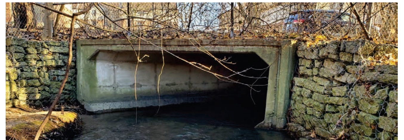
Example of Enclosed Watercourse in Storm Sewer
