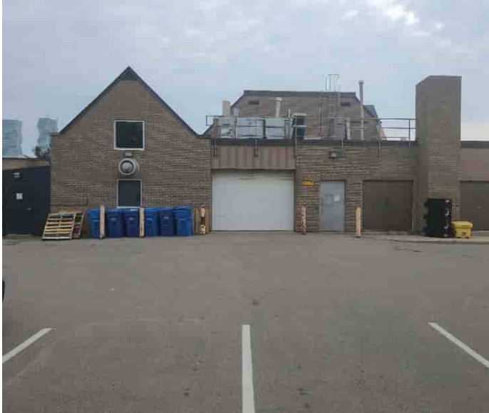
Image 1: Built up commercial/industrial structure and paved parking lot; no archaeological potential; image facing northeast
