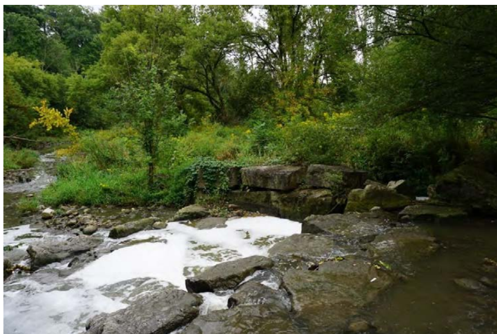
Photograph 9: View of Wolfedale Creek located in Study Area 2, the armour stone/rock retaining wall and the surrounding low-lying riparian area, looking southeast (AECOM 2023)
