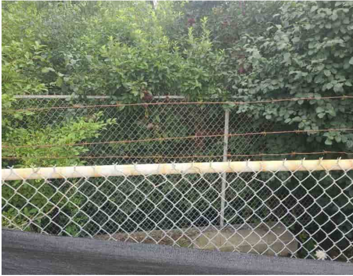
Image 5: Steep slope and concrete retaining wall; no archaeological potential; image facing east
