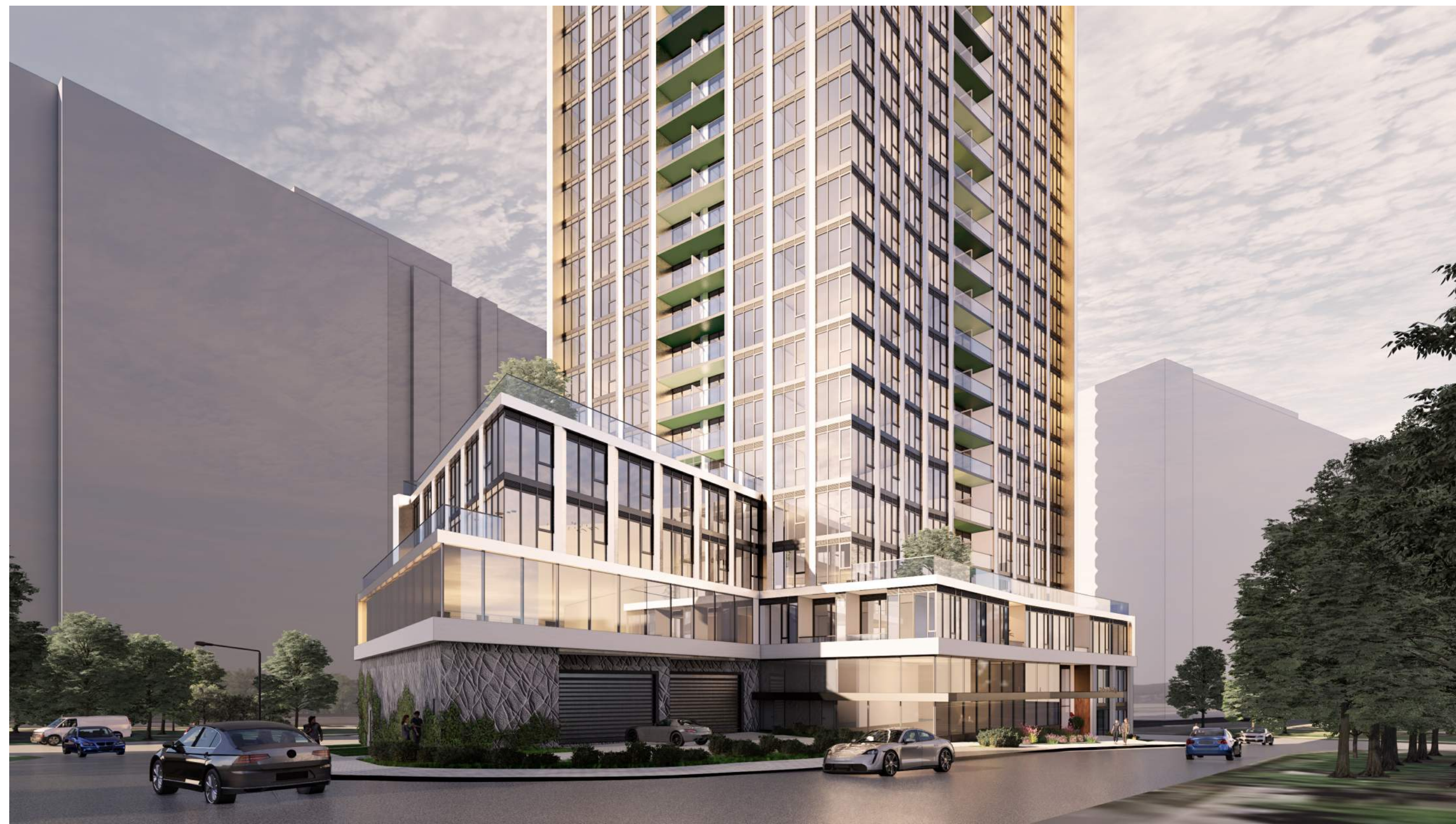
VIEW FROM CORNER OF KANEFF CRESCENT AND OBELISK WAY
