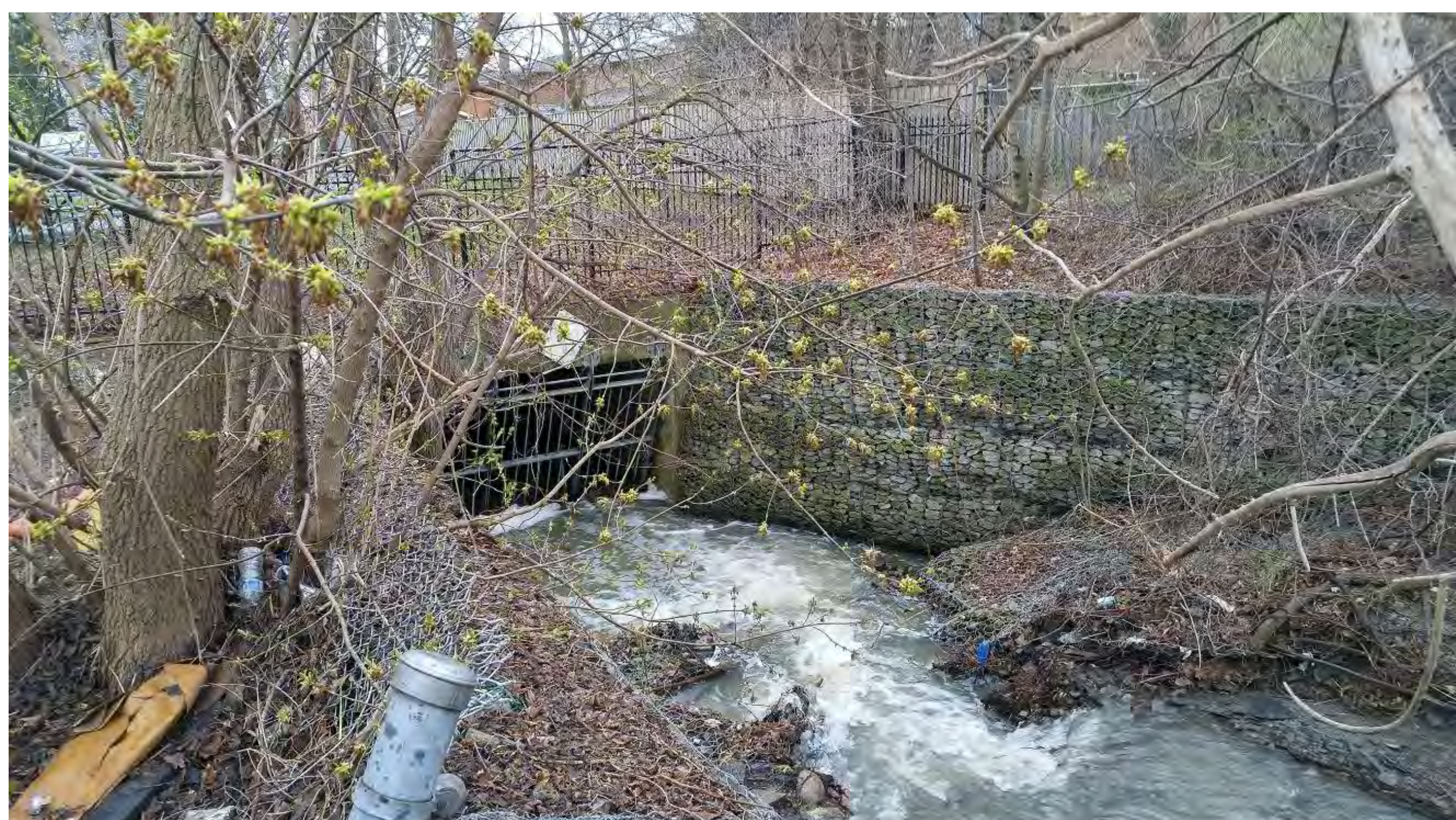
WATERWAY AT BACK OF SITE
