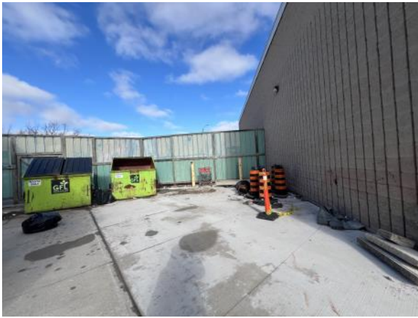
Photo 19: View of the waste bins at the adjoint barrier between Site Building A and Site Building B. Photograph taken facing northwest.
