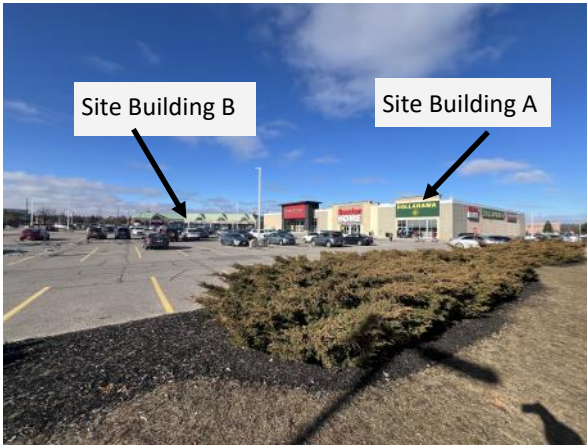
Photo 1: View of the Site buildings (A & B) on Phase One Property. Photograph taken facing northwest
