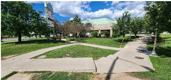
Image 3: Sidewalk and walkways, west edge of subject property, facing northeast.
