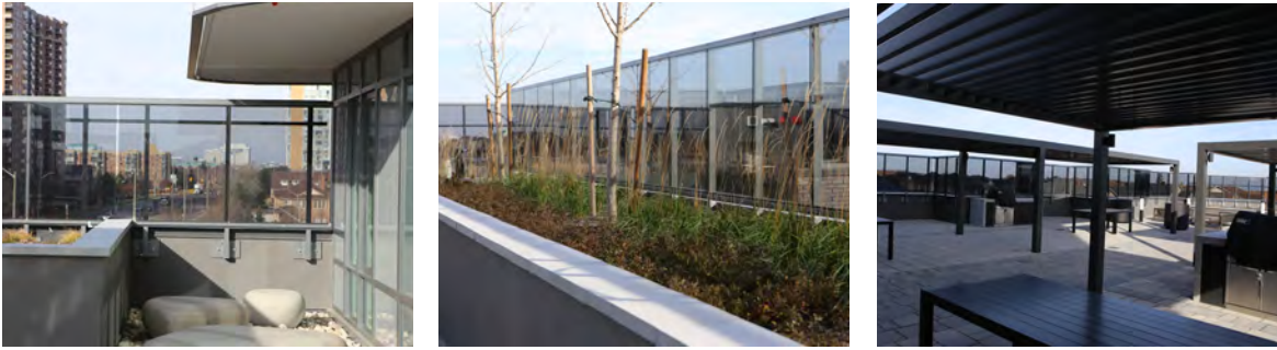
Examples of Wind Mitigative Measures at Activity Spaces (wind screens, raised planters, trellises)
