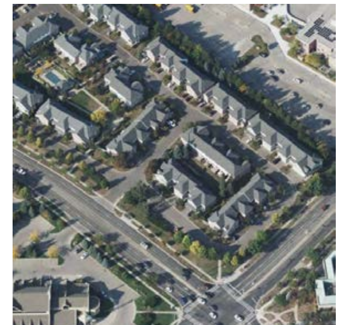
Low-Rise Residential Neighborhood at Glen Erin Drive and Erin Centre Blvd
