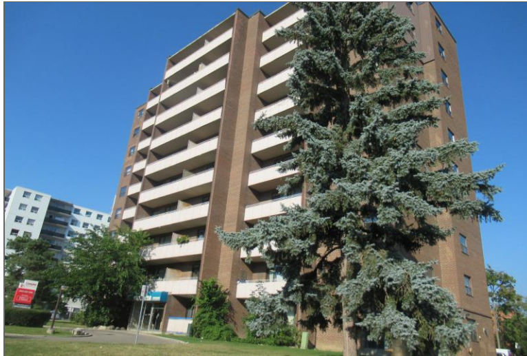
Photo 1 – Southeast elevation of the Site, looking northeast.
