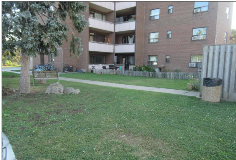
Photo 2 – Northwest elevation of the Site, looking southeast.
