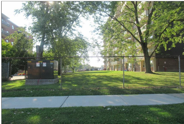
Photo 6 – Adjacent properties to the northwest.
