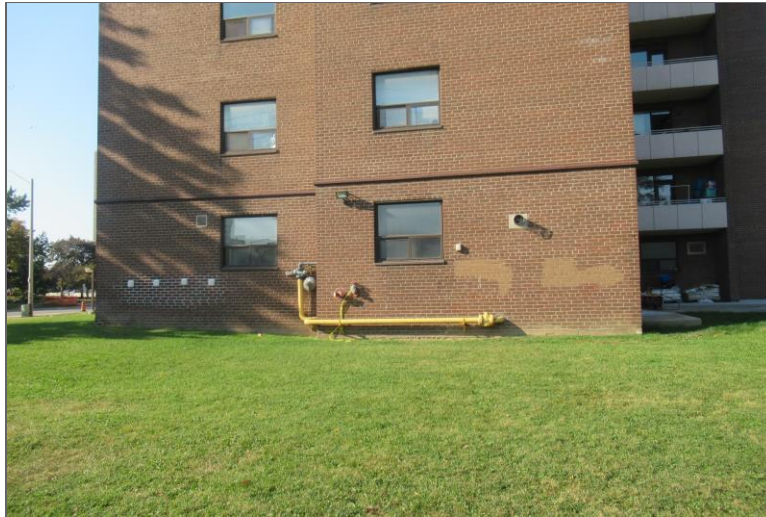
Photo 3 – Northeast elevation, looking southwest.
