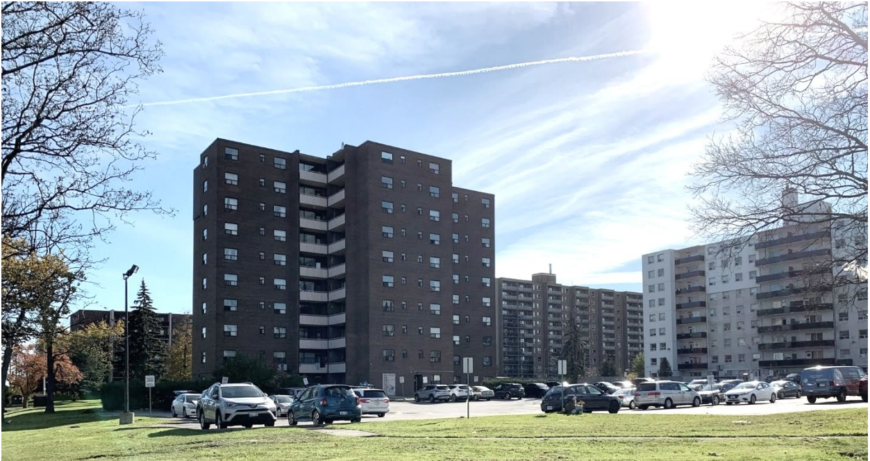
Figure 2: View looking southwest at the rear of the existing building.
