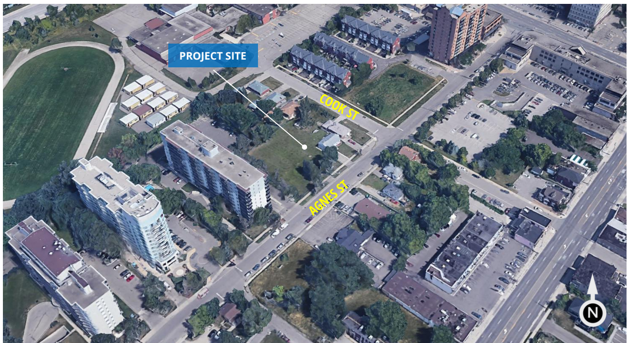
Image 1: Aerial View of Existing Site and Surroundings (Photo Courtesy of Google™ Earth)
