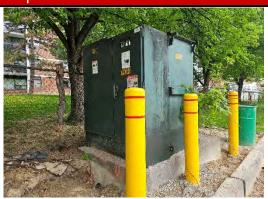
**Photo #8:** An oil cooled transformer located on the northwest portion of the Site.
