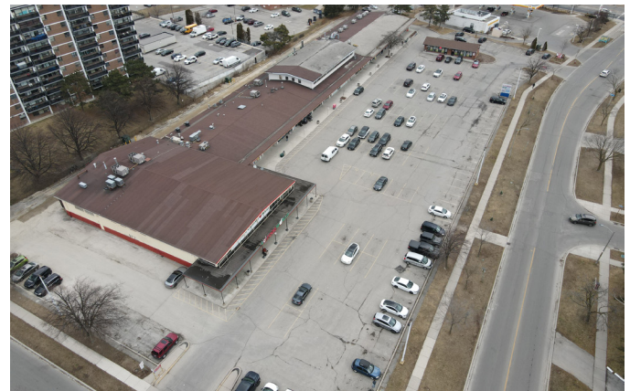
Figure 2 - Existing site conditions
