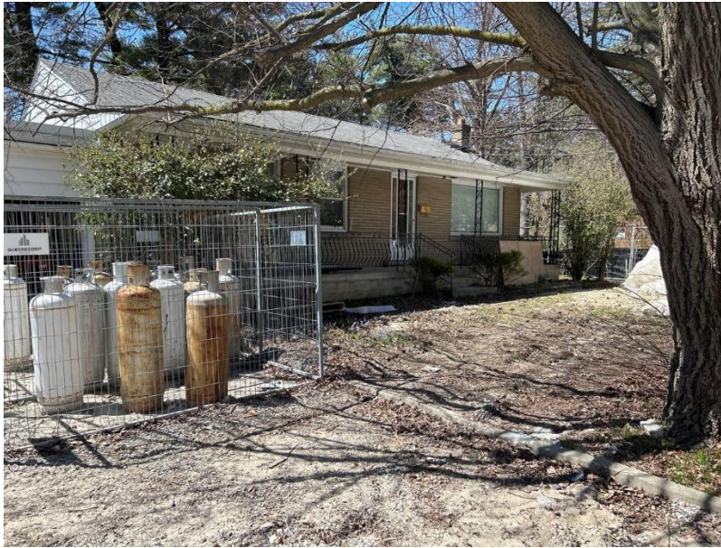
Image 1: View of the front of the house at 1154 Mona Road in the northeast of the subject property.
