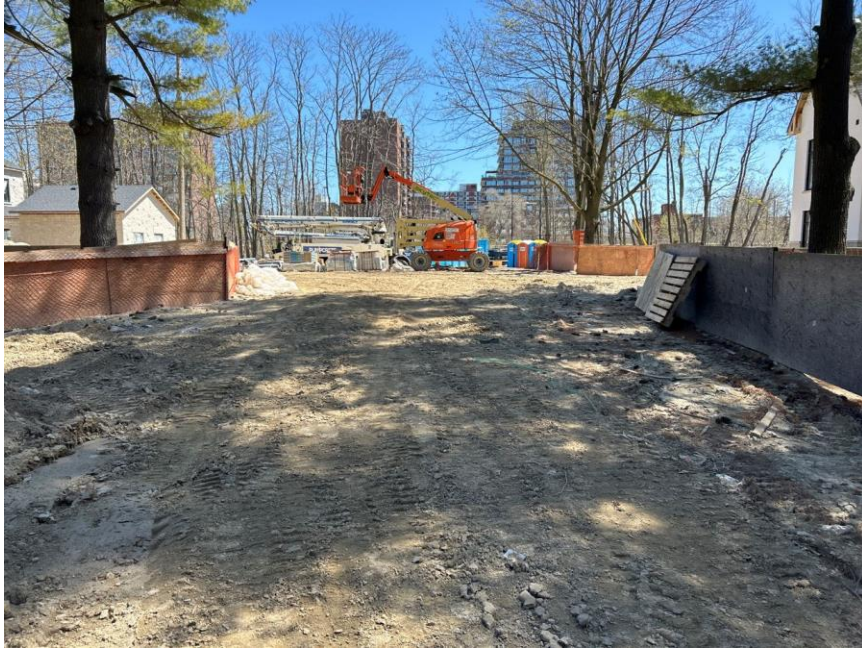
Image 3: View of extensive grading through the south of the subject property.
