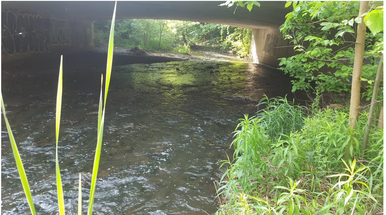
Photo 4: Slope Area at Section J-J' (looking south)
