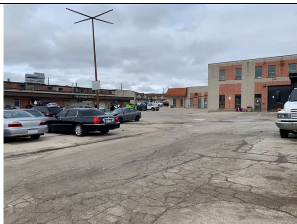
IMAGE 11 CONCRETE PARKING LOT AND TWO-STOREY STRUCTURES
