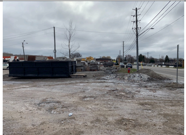
IMAGE 14 GRAVEL AREA WITH TEST PITTING AREA ALONG ROADSIDE
