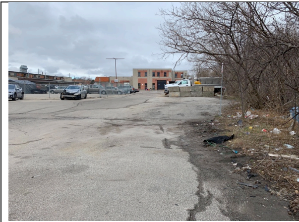
IMAGE 7 CONCRETE PARKING LOT AND TOP OF SLOPE
