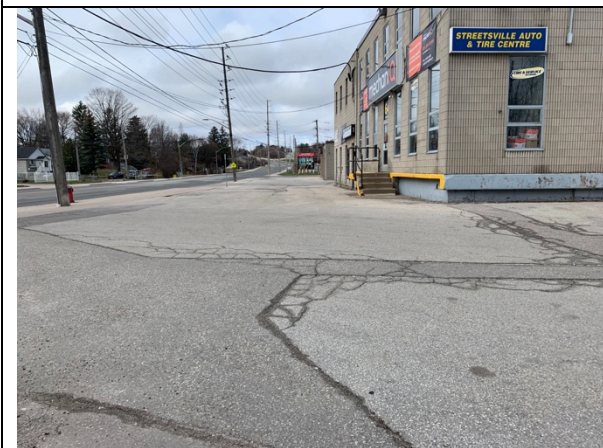
IMAGE 5 CONCRETE PARKING LOT/DRIVEWAY AND MECHANIC SHOP
