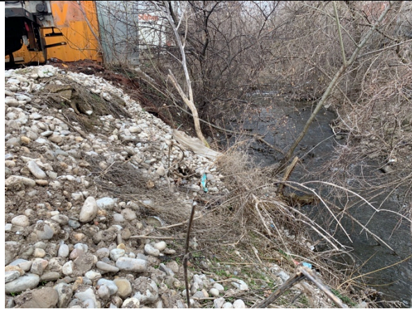
IMAGE 9 ROCK PILE AND STEEP SLOPE
