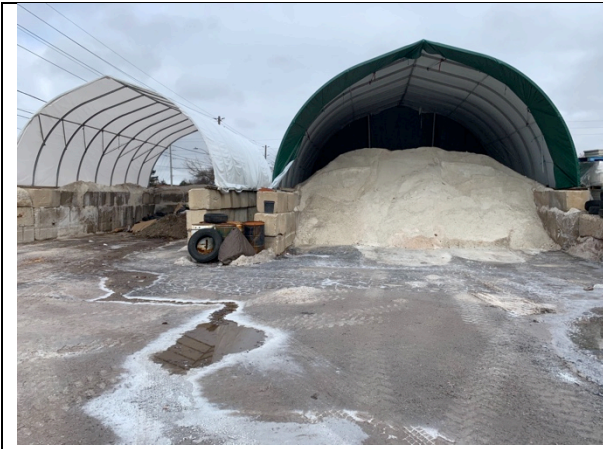
IMAGE 13 COVERALLS WITH CONCRETE FOOTINGS
