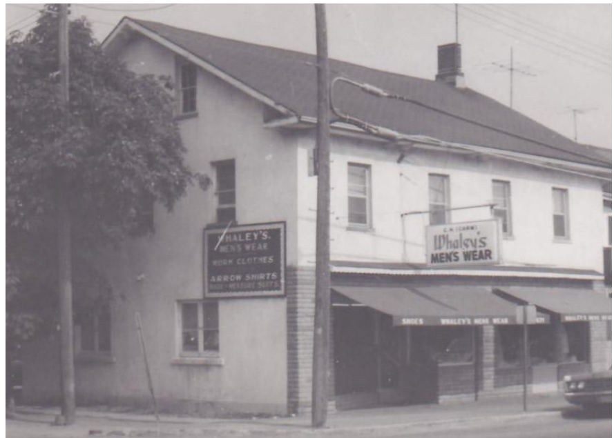
Historical image of 213 Queen Street South (photo credit: Streetsville Historical Society).
