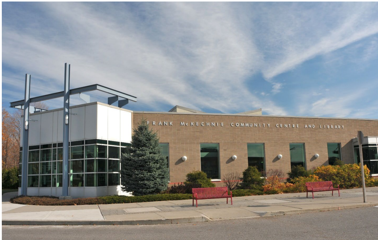
Frank McKechnie Community Centre
